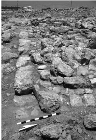
Figure 3.6d. Southeast corner of Wall 6005, looking west.
